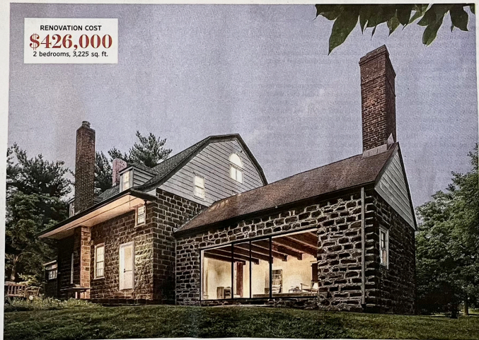
In the original portion of the house, part of a stone wall was replaced with a large glass window and french doors to provide light and views.
