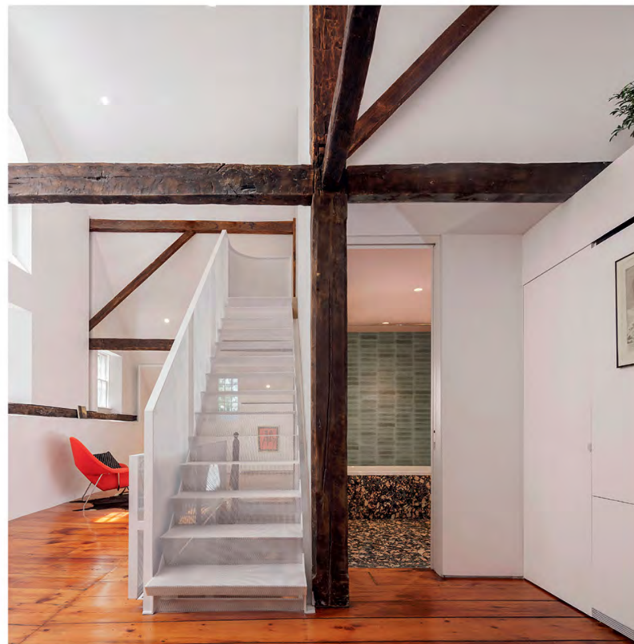
Views of the new staircase connecting the first floor and the attic, formulated as a pale volume with a parapet and steps in perforated steel, supported by a metal structure of minimal thickness.
